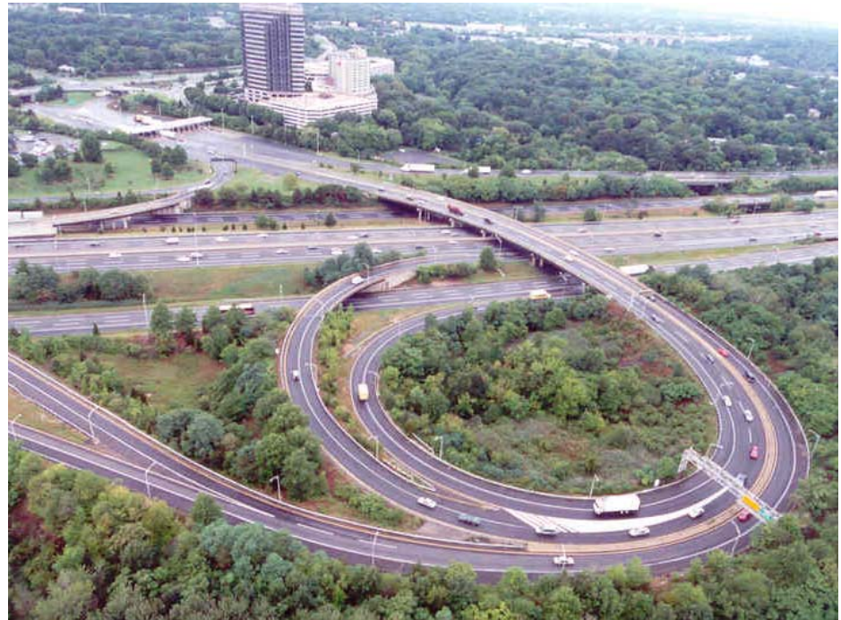
Figure 2. New Jersey Turnpike Entrance Ramp
