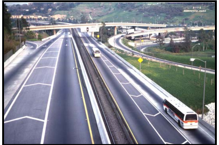
Photo Courtesy of HOV Interactive 2.0 I-10 (EL Monte) Bidirectional HOV Facility
