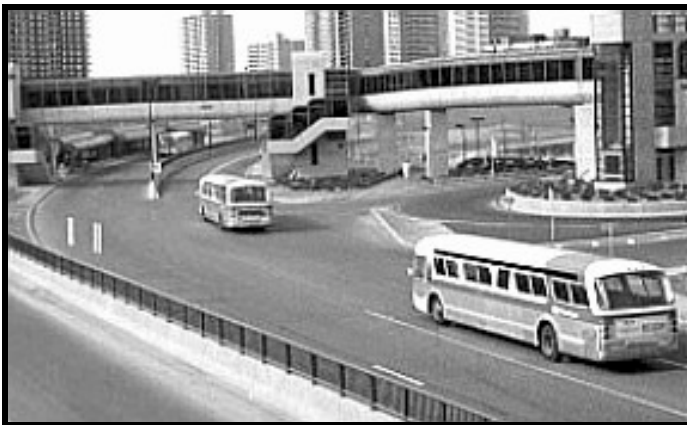
Example of Busway
