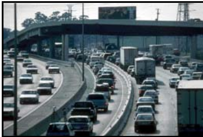
The HOV Lane on the Katy Freeway in Houston
